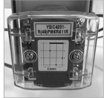
(3) 보호카바 부착된 모습 (Completion of protection cover attached.)
